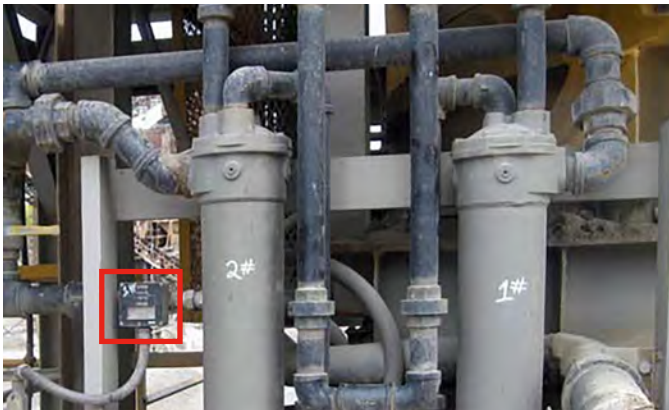
Model 816BC Flow Switch mounted on lube oil circuit for rock crusher at plant in Maryland.
