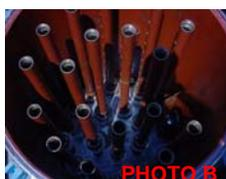
does not begin until after 12 — 18 months, so a yearly drain of the system will keep the bacteria from growing. Photo A is an example of a system that was not completely drained in over three years. It took a Kaydon Field Service Engineer a full day to clean out the water removal filter vessel (Photo B — holddowns & elements not shown).
